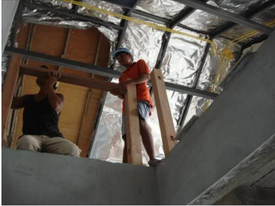
In villa F1 they are working with the fence.
