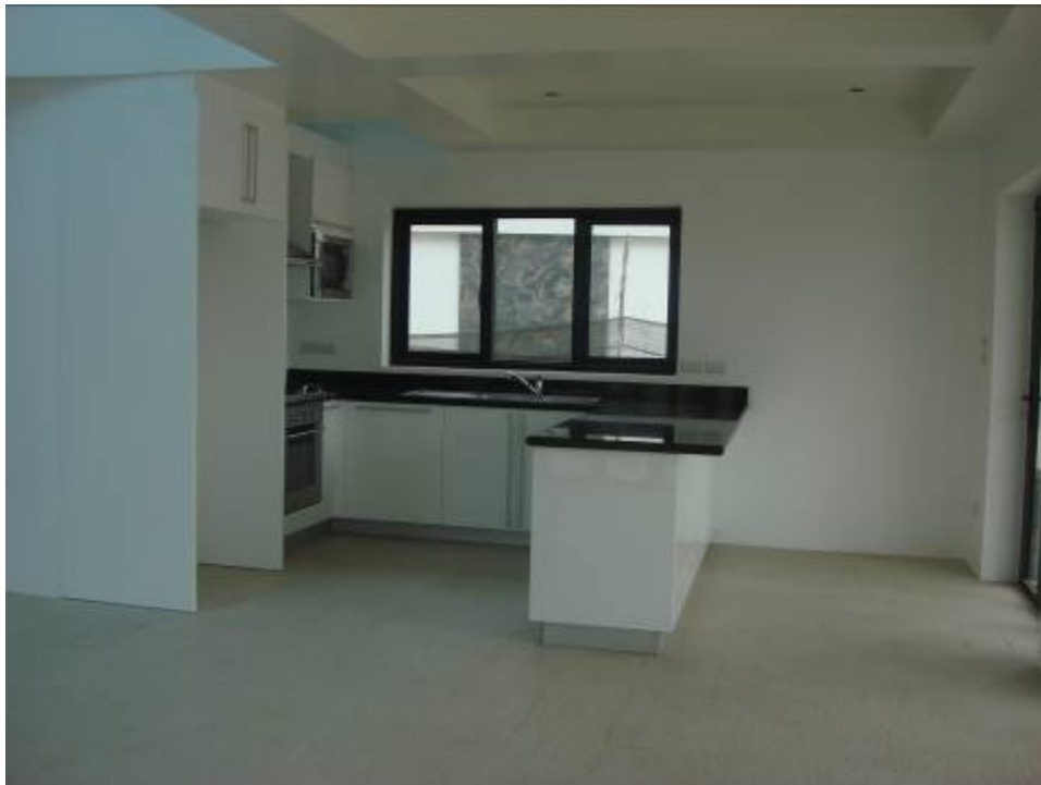
E2 Kitchen has been installed
