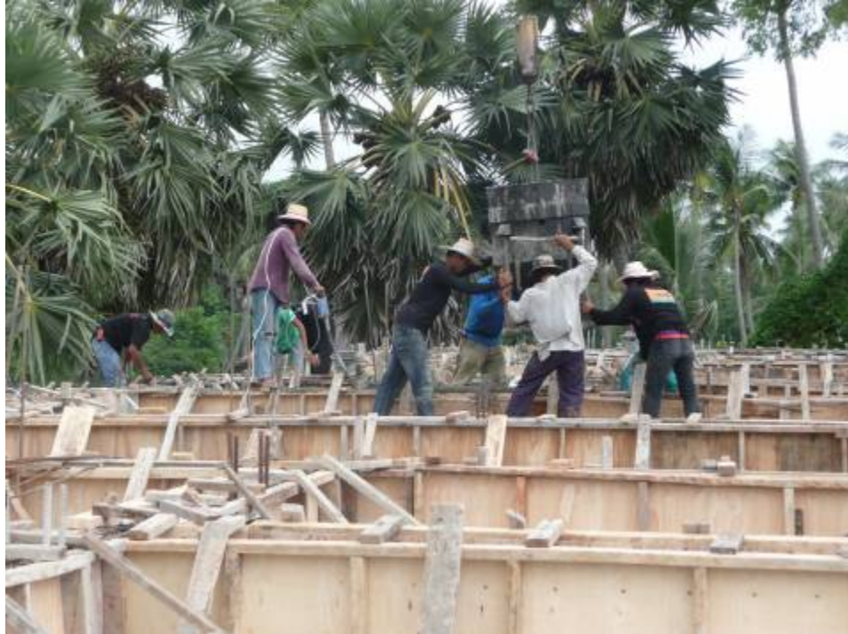
Workers at the beams on third floor Apartments
