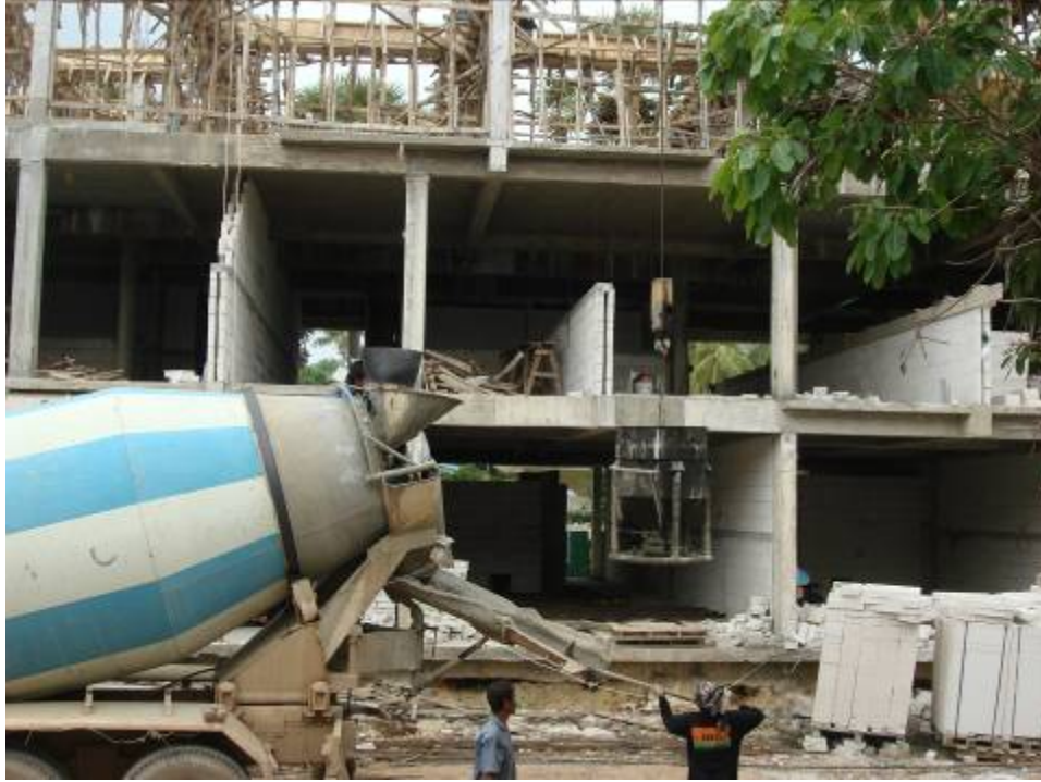
Concret Truck on site.
