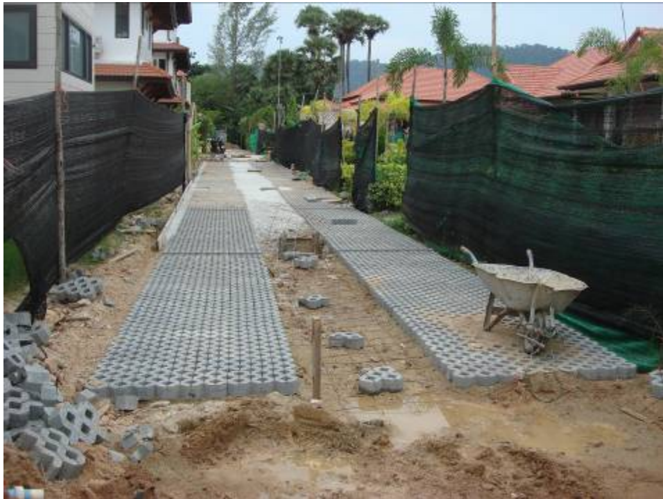
Slowly the last road on phase 1 is getting finished
