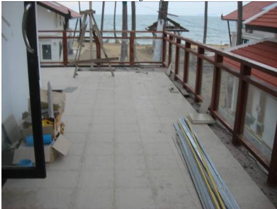
Villa F2 is getting tiles
