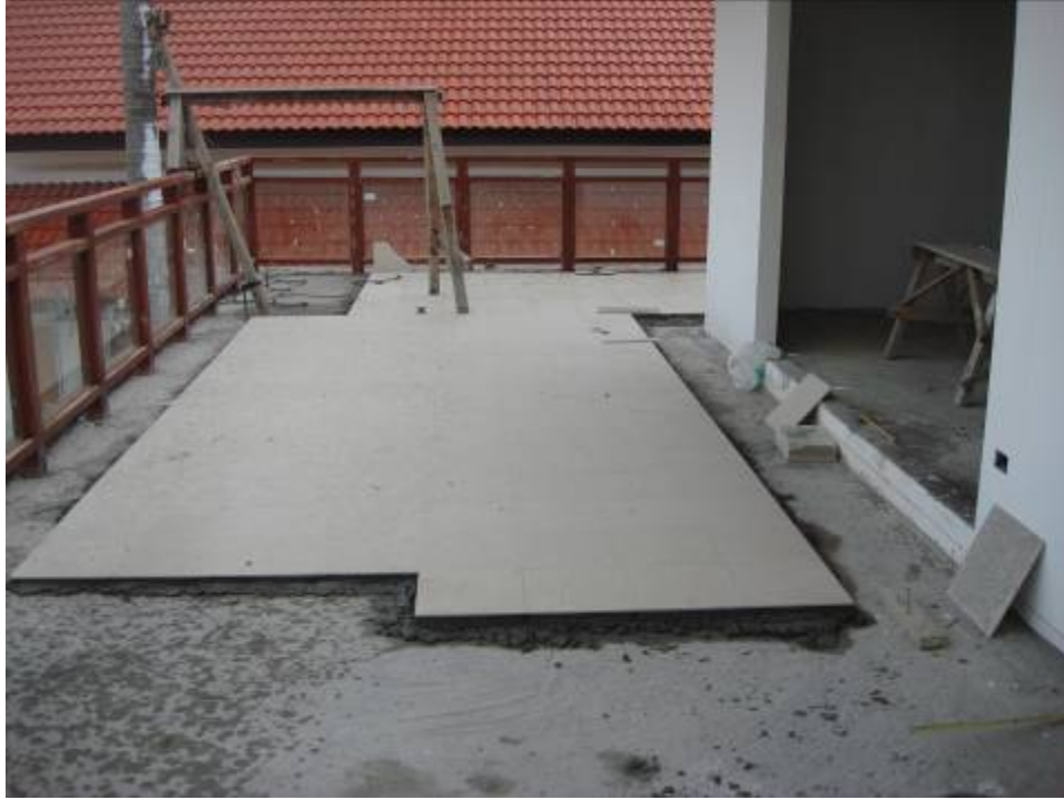
Villa F2 is getting tiles
