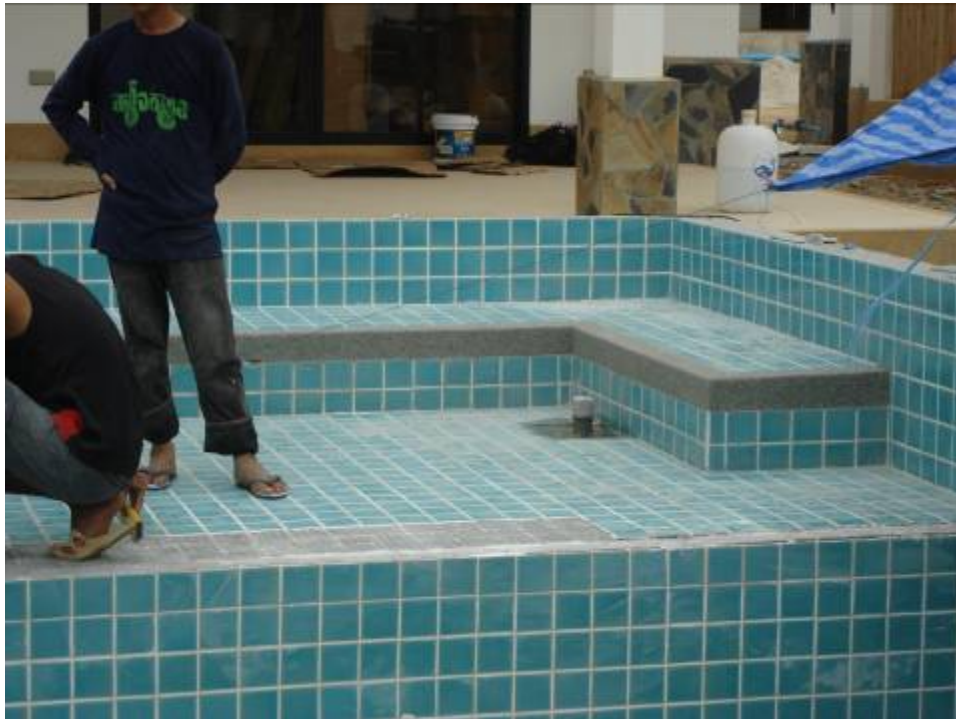
Swimming pool E7 is soon to be finished
