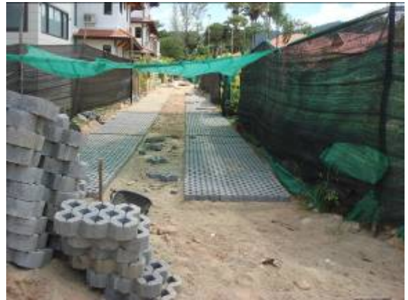
Last soi at B1-D1 is in finishing state
