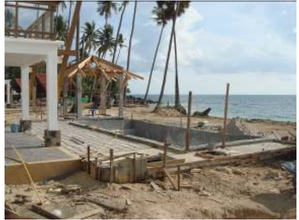
Villa E4 Pool and Sala is in progress
