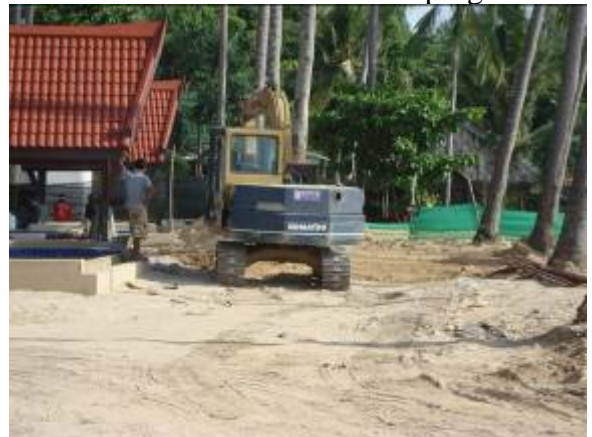
Villa E2, E3 preparation for putting grass
