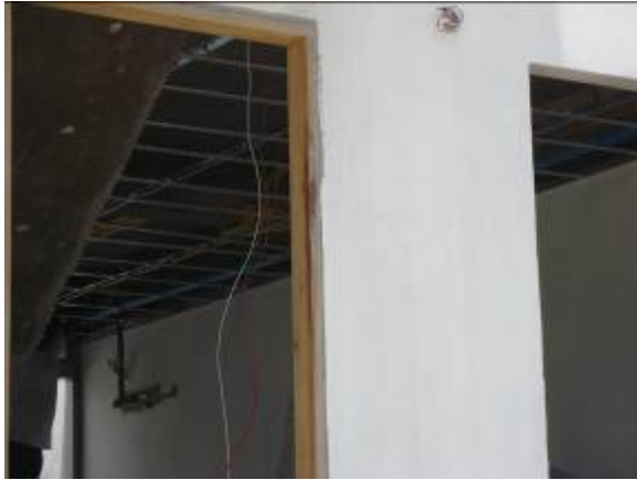
Electricity preparation in the Row house
