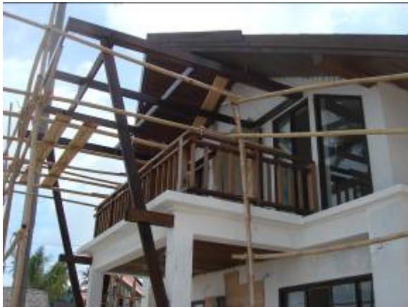
Painting work at villa E9
