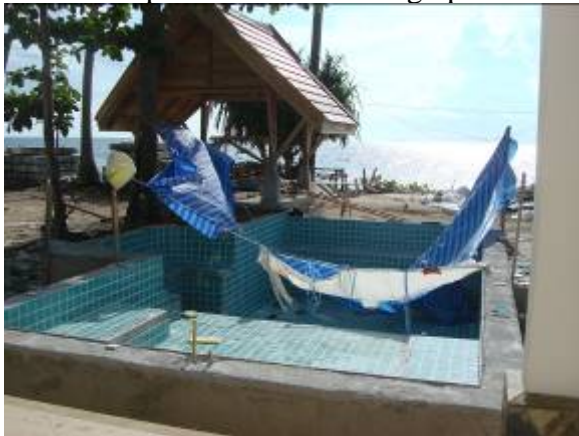
Villa E7 pool is getting tiled
