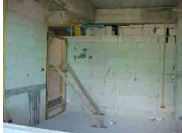
The woodframes is getting installed in the apartment building.
