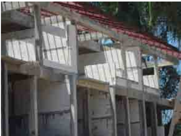
More walls are coming up at 3rd floor.
