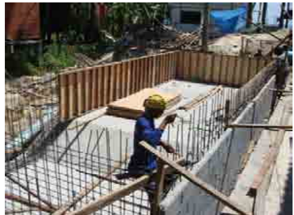
Villa F1 Swimming pool has started.
