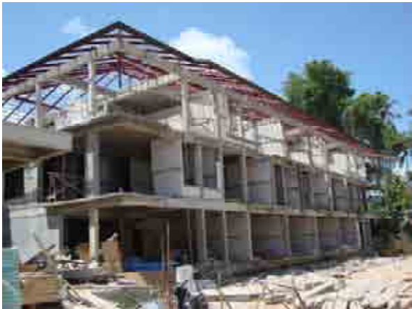
Roof Construction in progress. The Eveboard is installed on Apartment building.
