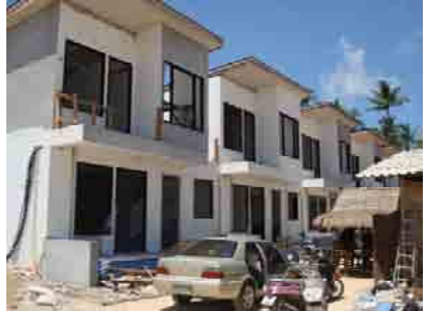
Fence on the row house is getting installed.
