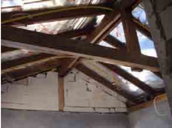
Ceiling and electrical work in F4 Small villa
