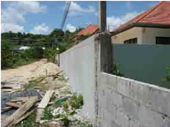
Plastering work at the wall at villa C12
