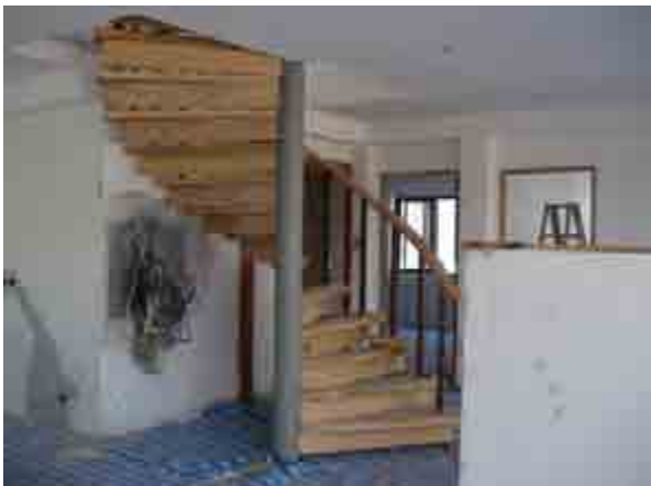
Stair work in villa F2
