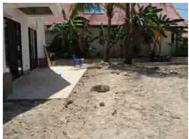
Outside leveling behind villa E9.
