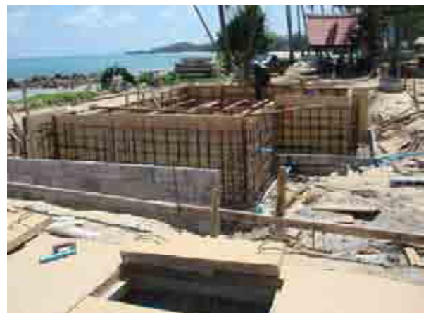
Villa E5 pool is in progress
