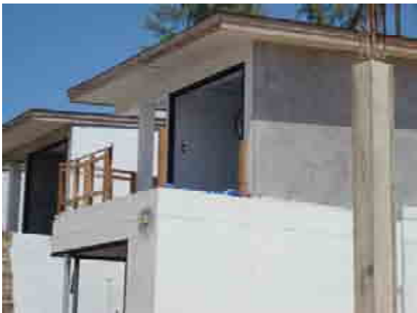
Fence work at Row house H105
