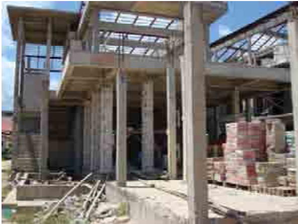
Cafe building columns has been bricked
