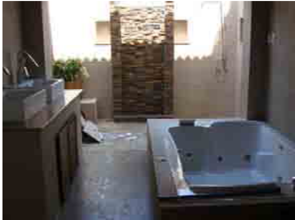
Small work left to do in villa E9. This is the bathroom.
