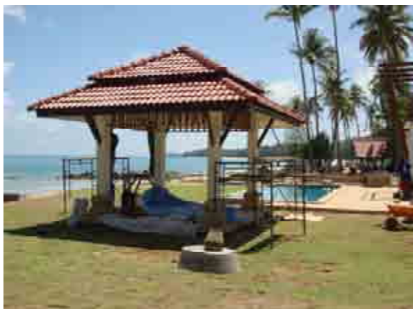
CaVilla E4 Sala is in progress
