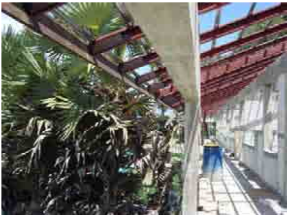
Walkway 3rd floor
