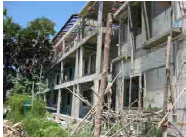
Plastering progress on the backside of the Apartment building.
