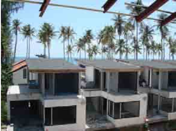
The row house is getting more tiles.
