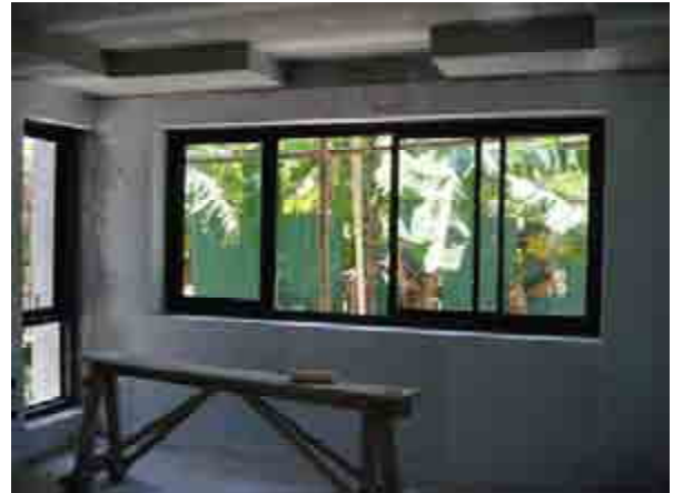
Villa F1 Ceiling work is in progress
