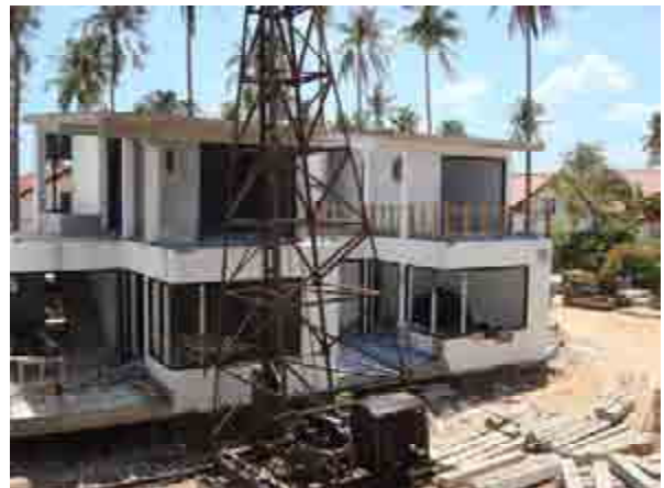
Piling machine and piles
