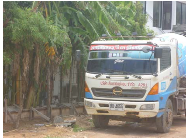
Wallwork at A7
