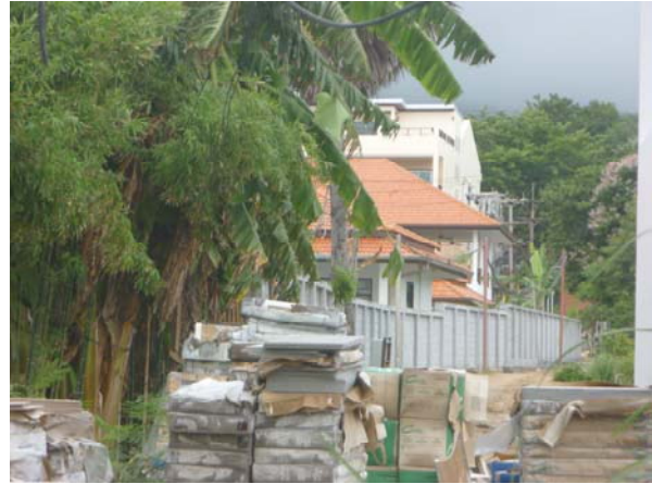
Wallwork at A7
