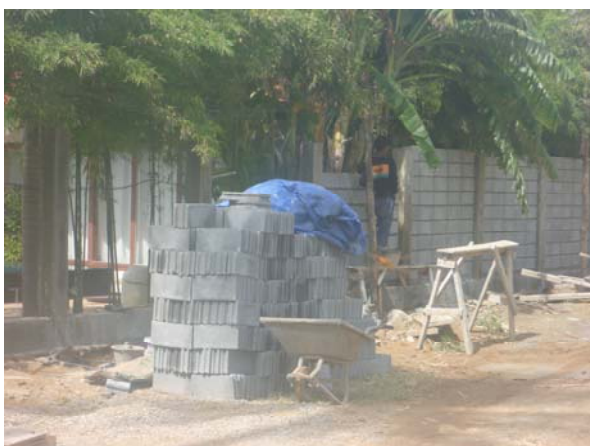
Wallwork at A7
