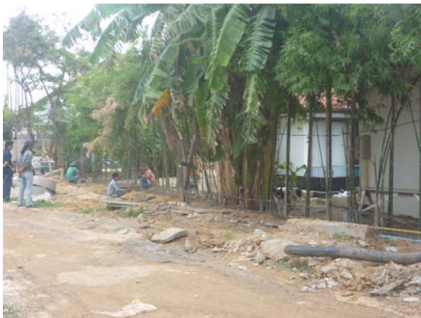
Wallwork at A7
