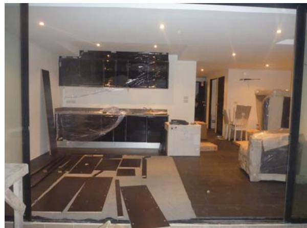
Installation of furniture in G101, G106, G201, G207
