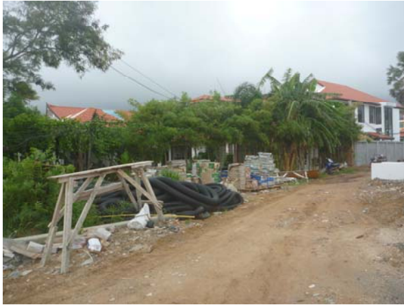
Wallwork at A7
