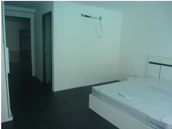
After installation G101
