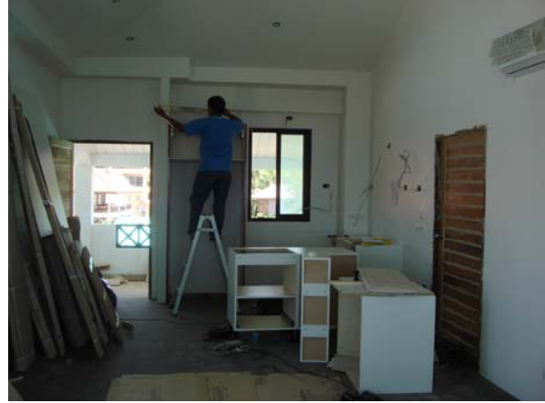
Installing of kitchen 301
