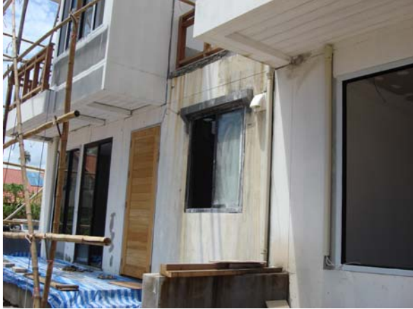
Doors and windows are installed in rowhouse H105
