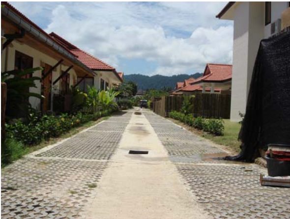
Planting bushes at phase. Soi between C1 and C8
