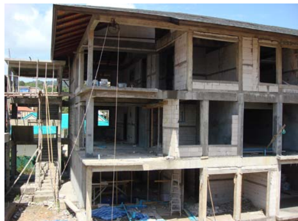
More walls are coming up at the Apartment building
