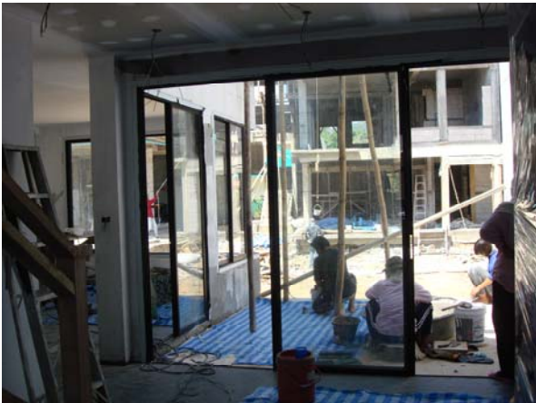
Sliding doors installation in rowhouse H105
