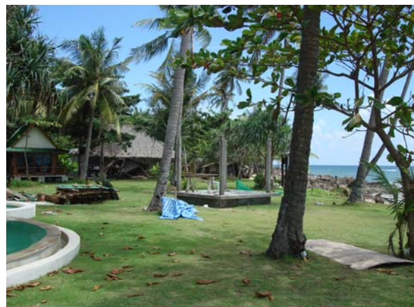
Sala work at villa E1 in progress
