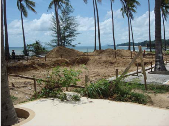
Pool E8 lined up and ready to start
