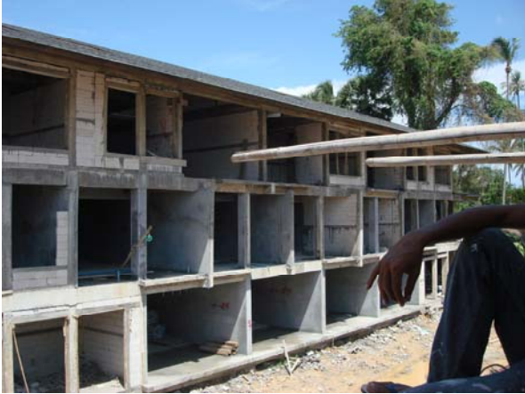
More plastering in progress inside the apartments
