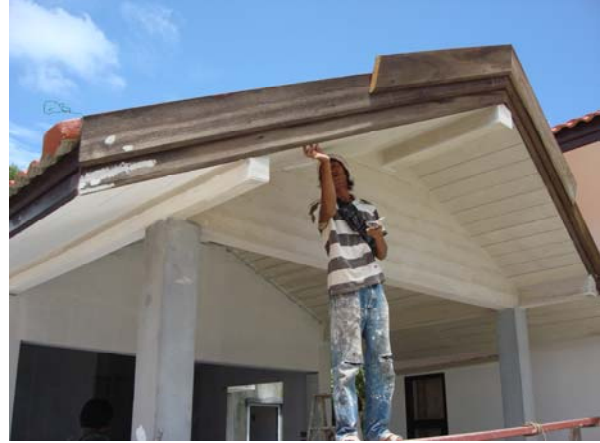
Painting work att F4 small villa
