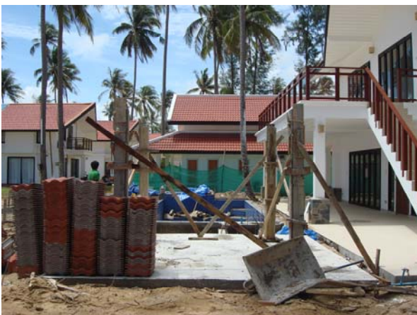
Sala work at villa F2 continues
