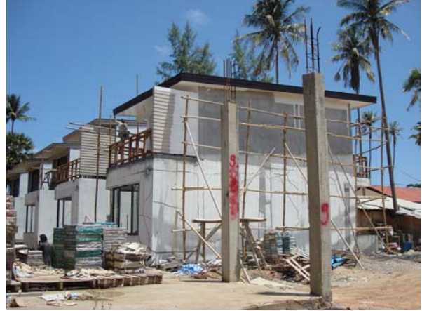
Balcony walls is getting installed at the rowhouse
