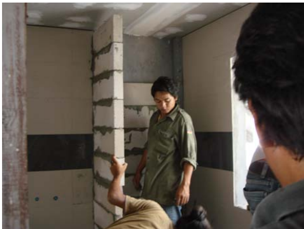
Bathroom work in F4 small villa
