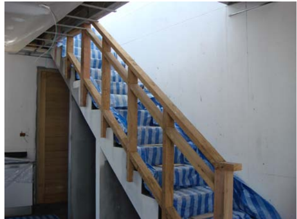
Fence ready to be painted in rowhouse H105
