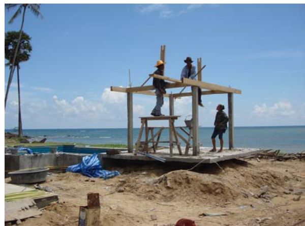
Sala work at villa E5
