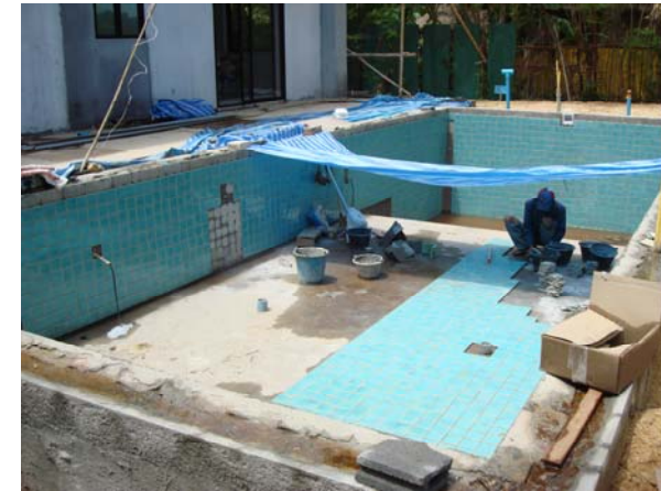
Tiling of pool F1 continues
