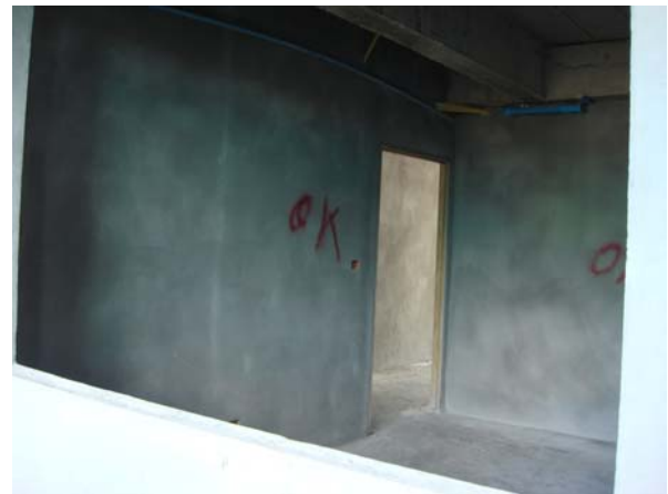
More plastering in the apartments This is G102 that is finished
