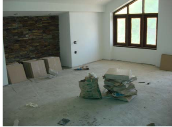
Tiling work at villa E5 about to continue
