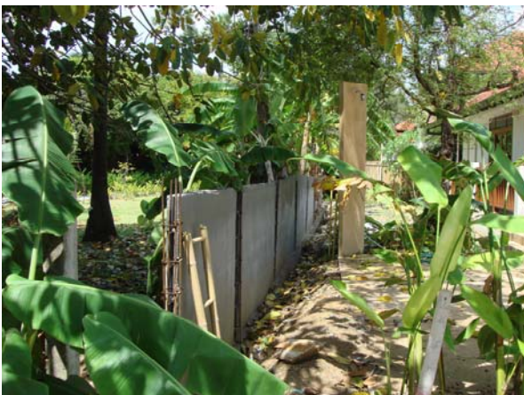
Wall work at villa A10
