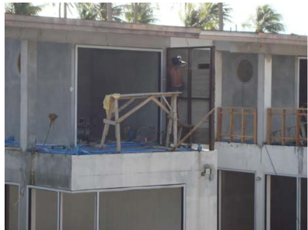
More balcony walls are coming up, now at H103
