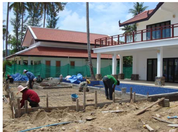
Poolarea at villa F2 in progress
