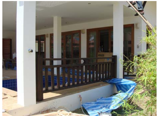
Fixing work at villa A9
