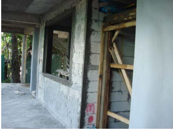
Door columns are beeing made
