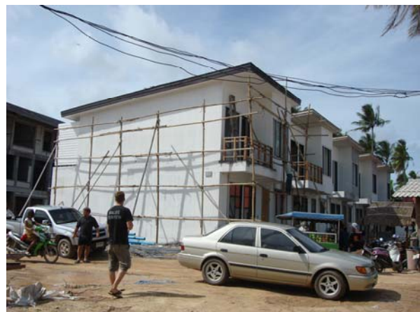
Painting work at the rowhouse
