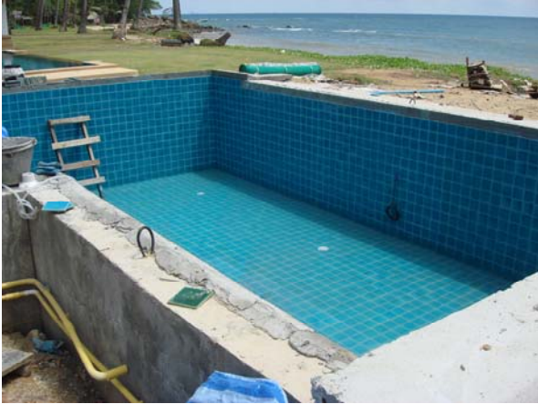
Tiling work almost finished at pool E5
