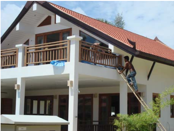
Fixing work at villa A9
