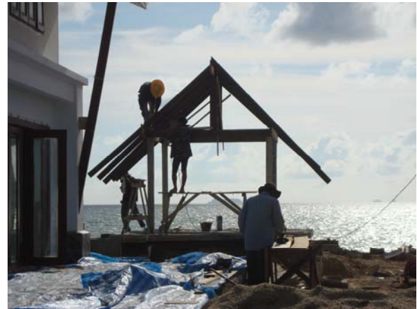
Sala work at E5
