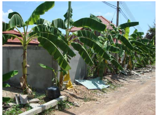
Wall at villa C12-C14 almost finished
