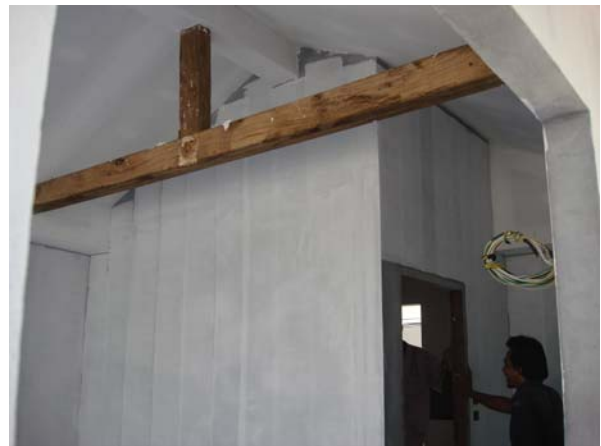
Ceiling work at F4 small villa
