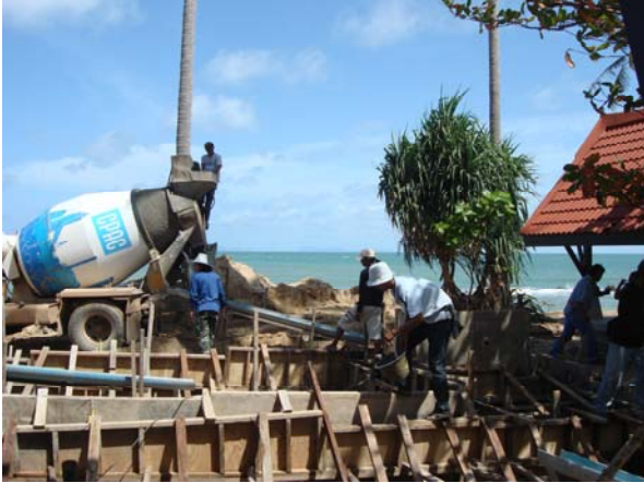
2009-07-25 Concrete for pool E6
