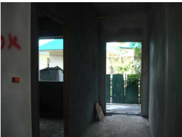
Painting work can soon be started in G102-G104
