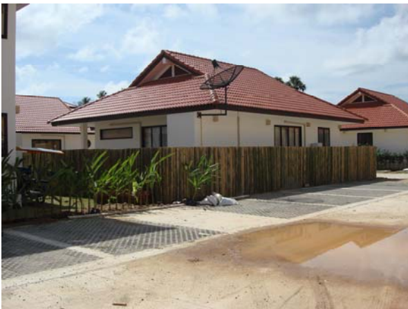
Villa C9 bambuwall. Picture taken from parking area
