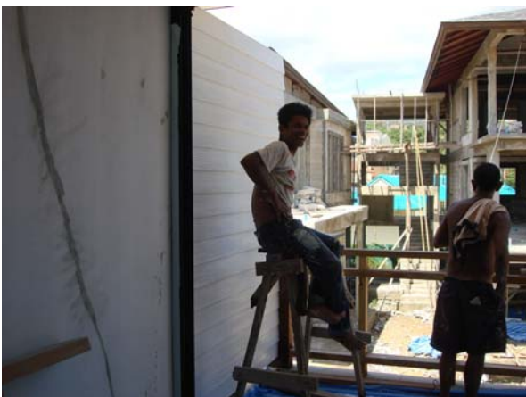
Wall work at balcony H105
