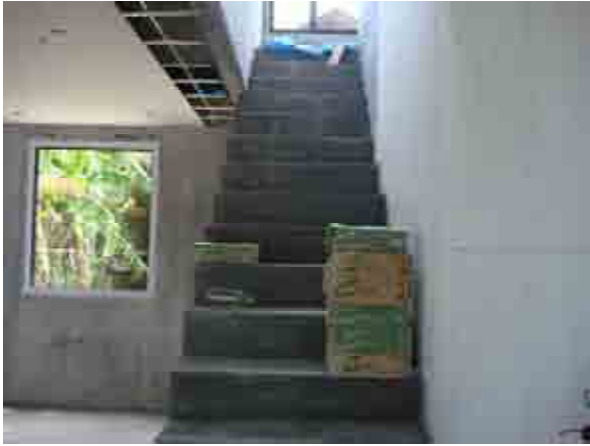
Stair tiled in rowhouse H102
