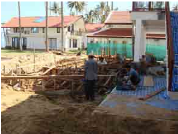
Pool work at villa F2
