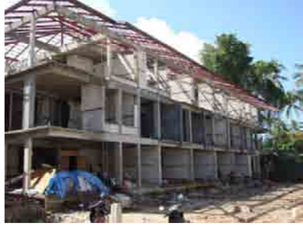
Apartment G202 & G203 have been plastered
