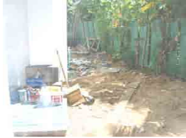
Fill up work at villa F2
