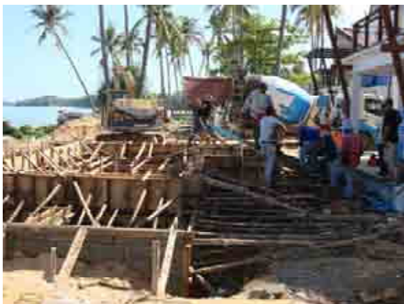
Concrete work at pool E5
