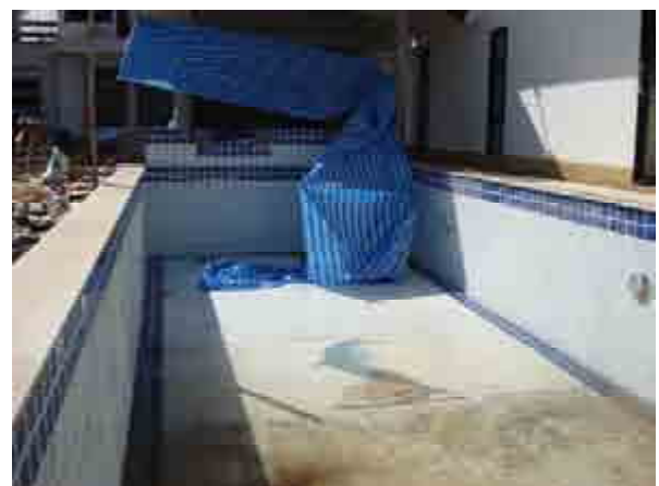
Dolphin installed in pool F4
