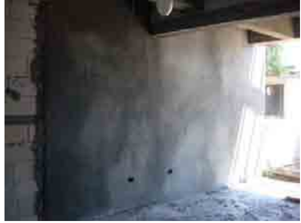
Plastering work in the apartments has started.
