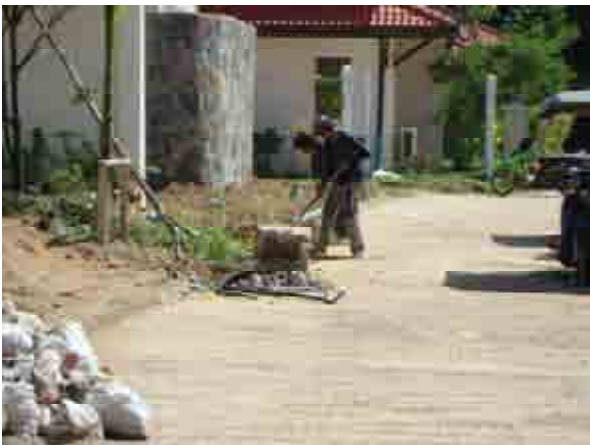
Covering pipes behind villa A3
