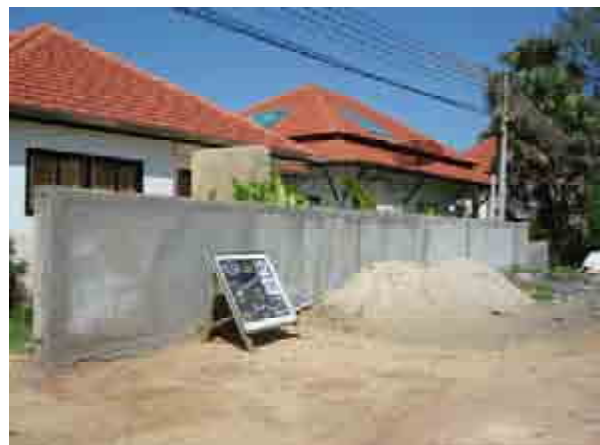
The surrounding wall at villa C6
