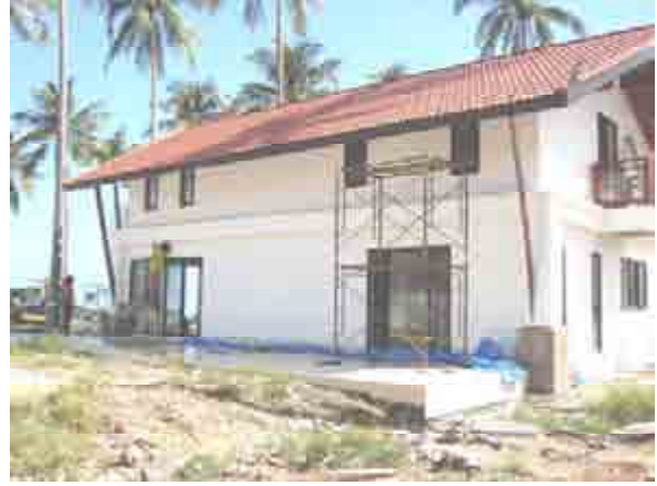
Painting work at villa E8
