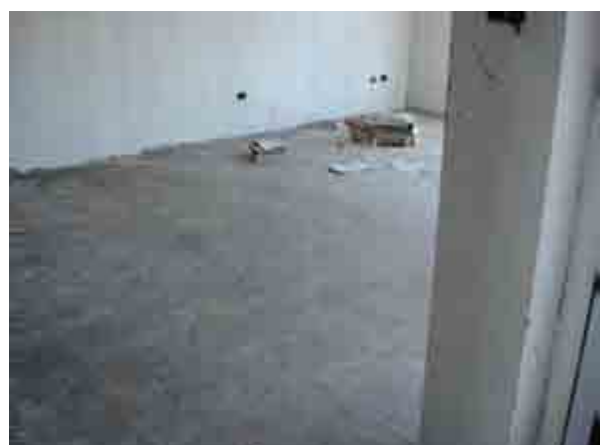
Tiling work in the row house H102
