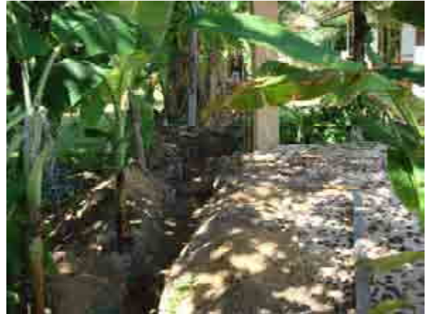
Wall work at villa A10
