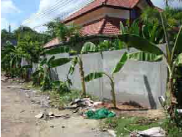
The surrounding wall at villa C12
